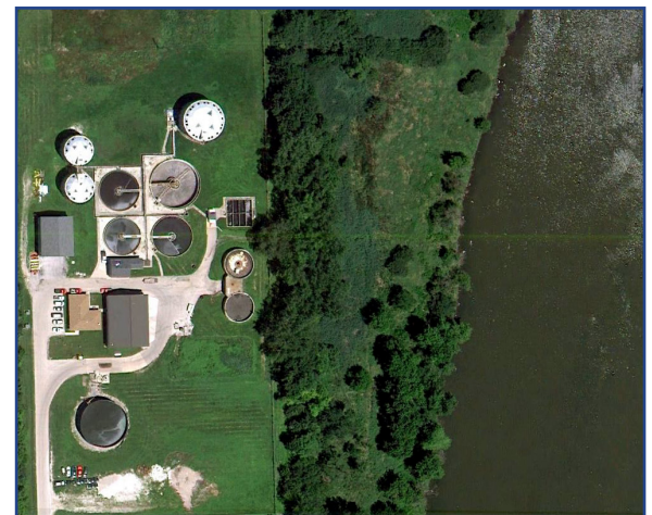
City of Crest Hill Eastside Sewage Treatment Plant
